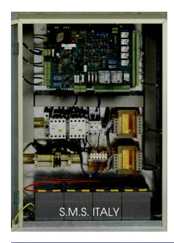
The E.M.R. device (ARD) is used in traction lifts, to assure the car return to floor and the door opening in case of main power failure.
