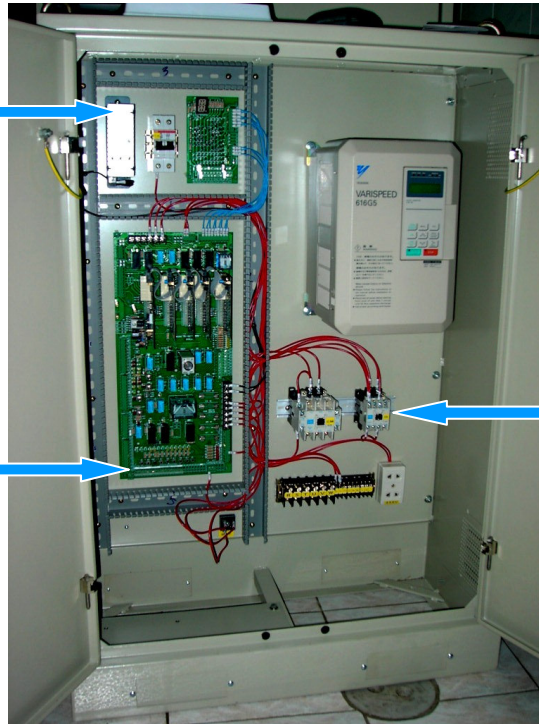
Magnetic contactor "Mitsubishi" S-N35, S-N11 Receptacle 220V and Power wires and Control Wires terminals
